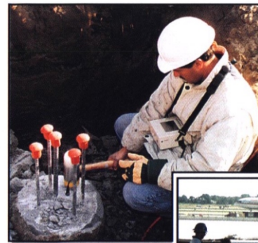
PIT testing of Augercast piles
