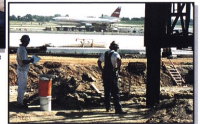
Monitoring pile driving
